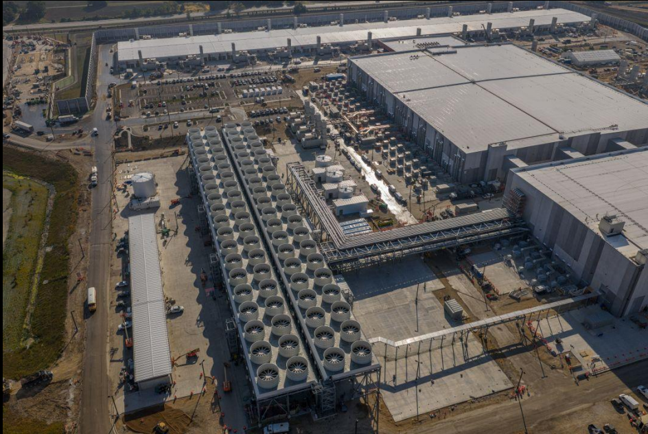
Microsoft's New Wisconsin Datacenter Campus
